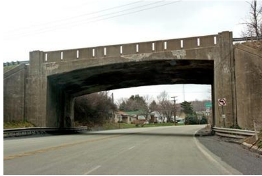
Fig.1. Stoystown Road Overpass (BridgeMapper, 2011)
